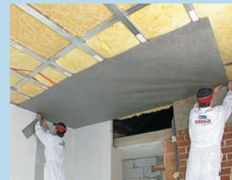
4 Namestimo parne ovire ( S_d \approx 2 \text{ m} ) ali parne zapore ( S_d \geq 100 \text{ m} )
